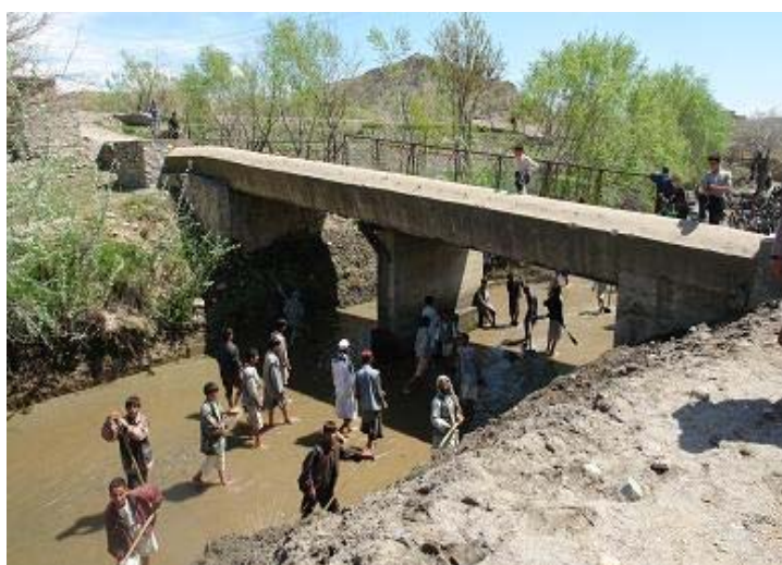
Rehabilitation and cleaning of canal in Mahmoud Raqi district as a result of DIAG compliance in Kapisa province.
