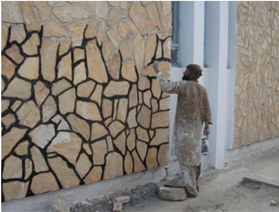
(Photo: Repair of Drug Rehabilitation Center in Jalalabad)
