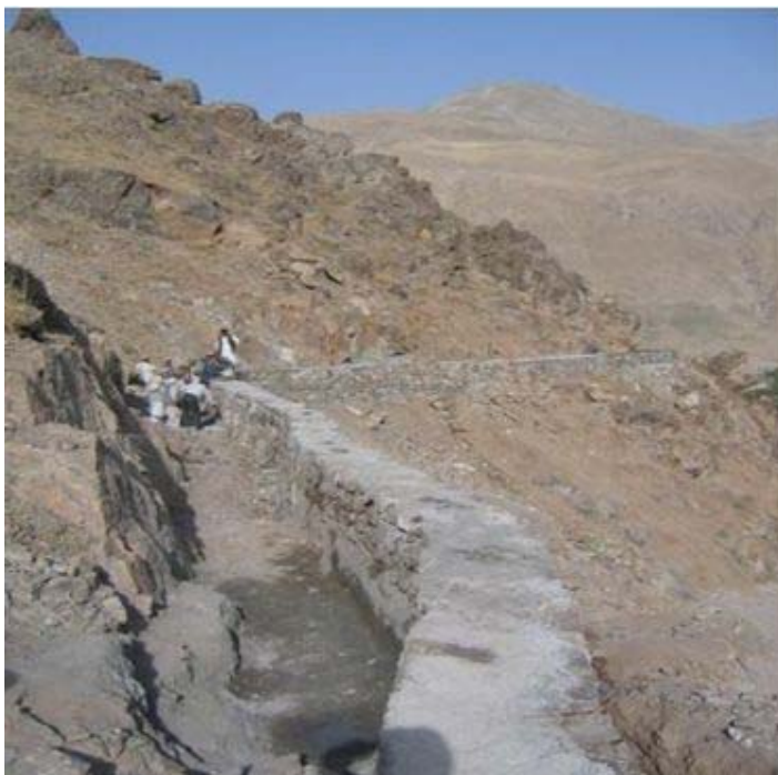
Picture 3: Construction of a water supply canal for the micro hydropower plant in Badakhshan.
