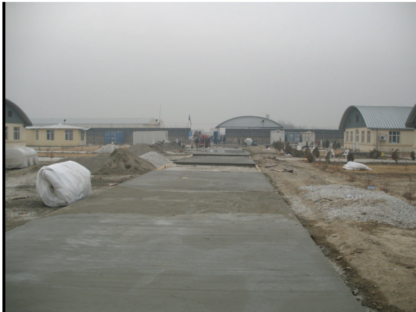
Construction on interior road and sidewalks at the IEC, January 2008
