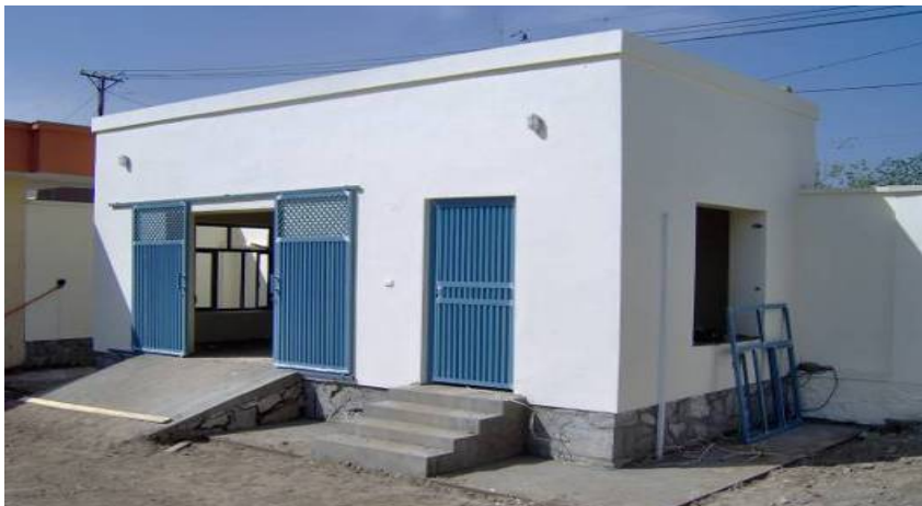
Photo: Generator room of Vocational Training Center, Nangahar
