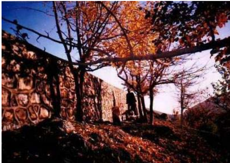
Retaining Wall in Chora District, Uruzgan Province, constructed by NABDP
