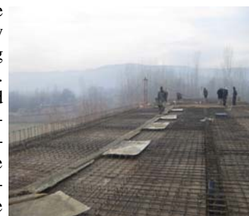
16 Class Room School Constructions in Zari District in Balkh
