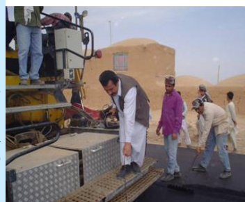
Chimtal District 16KM road asphalt activities
