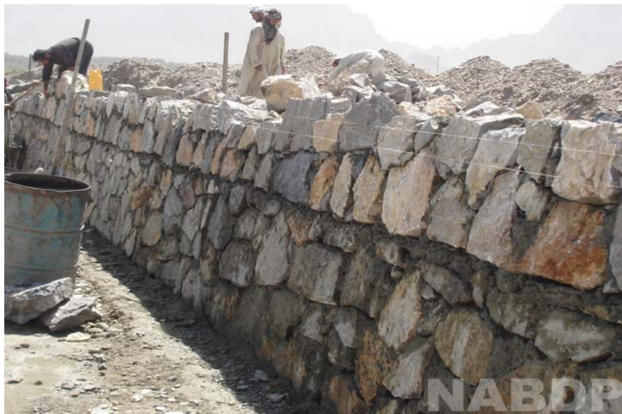
A community protection wall project being implemented in Kandahar
