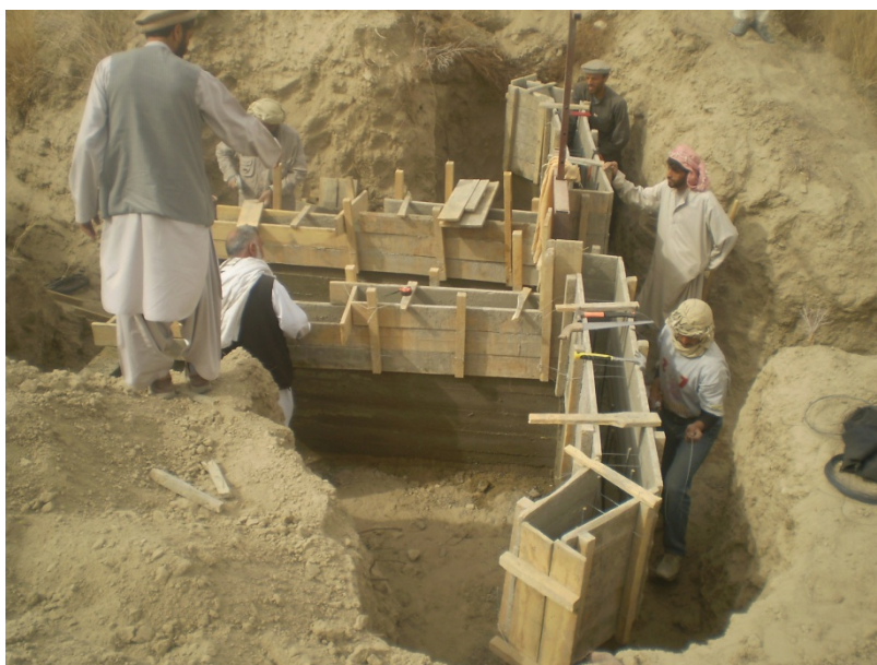
Construction of a water divider in Chakhansoor district of Nimroz province
