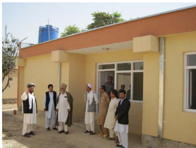
Baghlan Jadeed Primary court after completion
