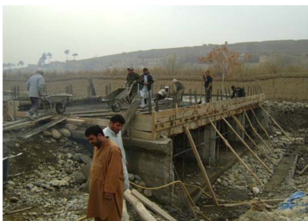
Bridge construction in Paghman district-Kabul province
